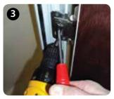
Secure the screws in the side plate.
