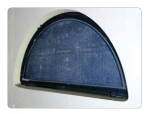
Lower the glazing panel into cassette. Ensure it is the correct way round. Push down gently onto sealant.
