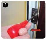
Lever the slide plate (B) with a screwdriver in the adjustment slot
