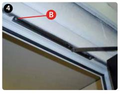
Fix frame-side of the restrictor to the outer frame using the remaining fixing screws at points B  $\&\,C.$
