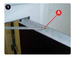
Fix leaf-side of the restrictor using the predrilled pilot hole at point A and one of the supplied screws.
