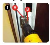
Remove the 2 screws that clamp side plate (B) to frame plate (A) to all three hinges
