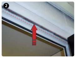
Open the restrictor and locate it in the bead channel of the outer-frame.
