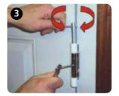
When in position secure the socket screw and replace the covers. Take care not to overtighten.
