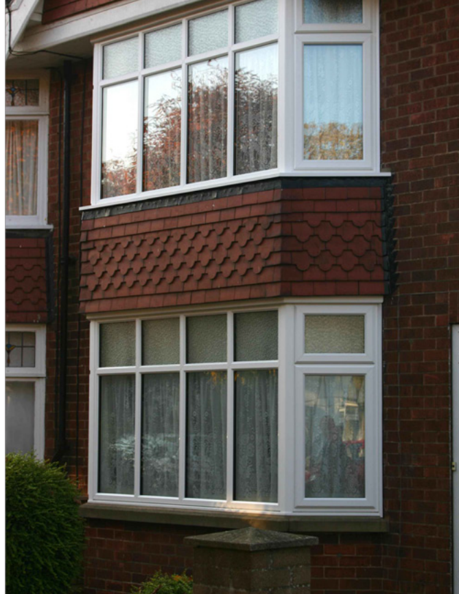
Structural Bay Window
