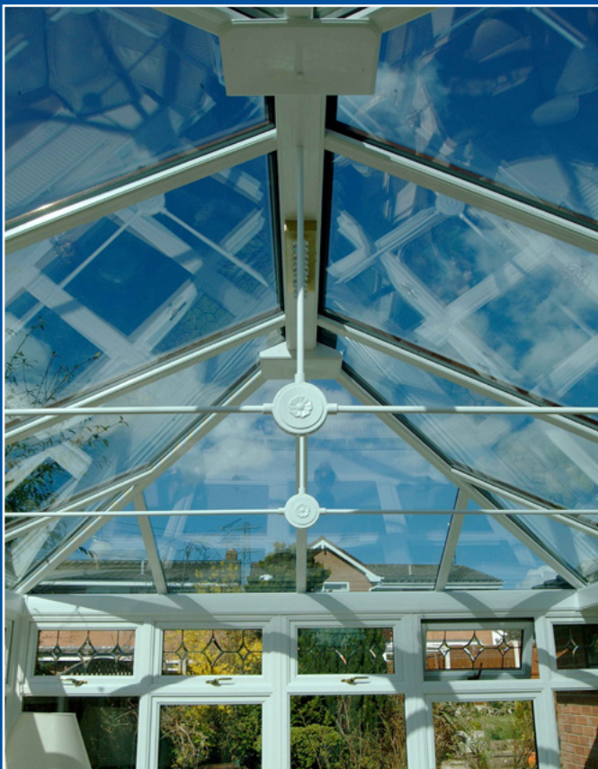
Anti-sun self cleaning glass roof
